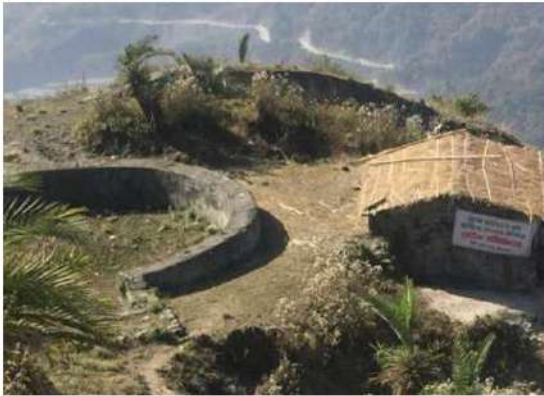
Photo 1 (Rainwater Harvesting Tank)
