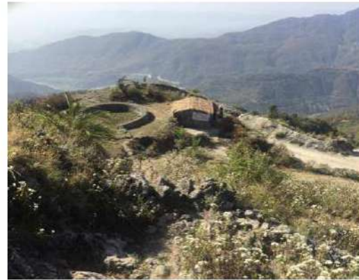
Photo 2 (Rainwater Harvesting Tank)
